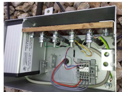
Layout of the Rail Module and the Trackside Box.
